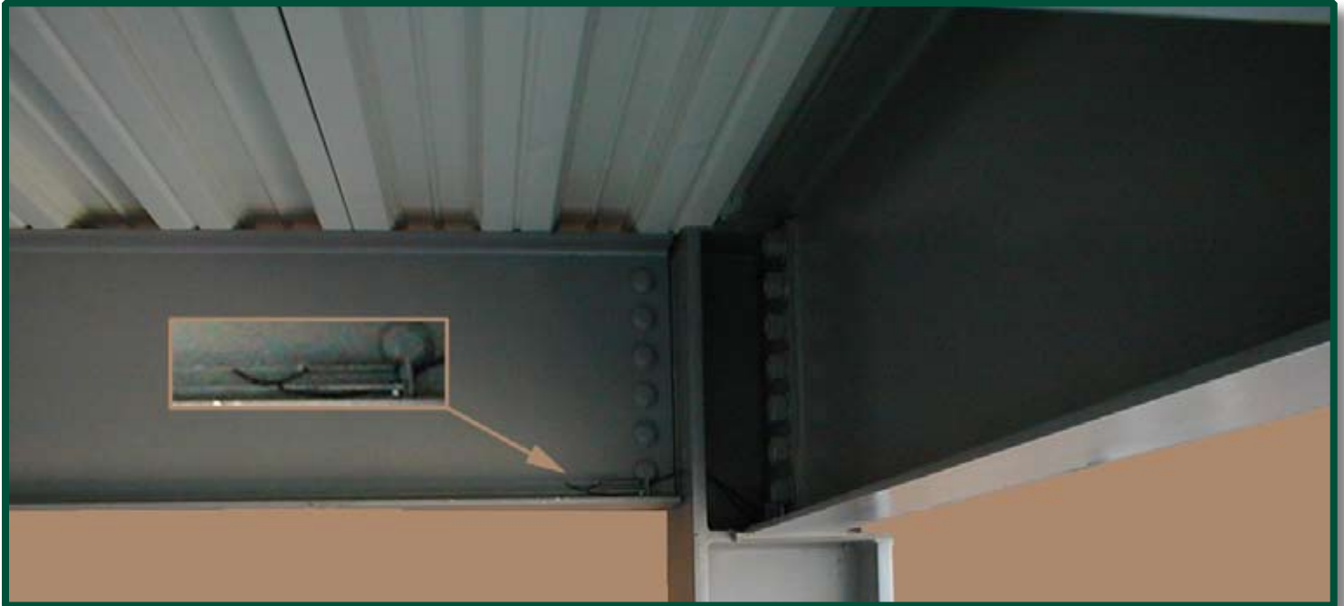
Stud Welded Insulators on I-Beam
